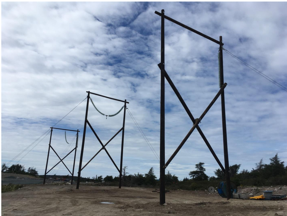
Figure 2 - Completed Wood Pole ERS at SOP
