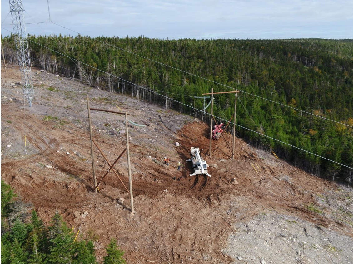
Figure 7 - Jumper Installation at Angle Deadend ERS.
