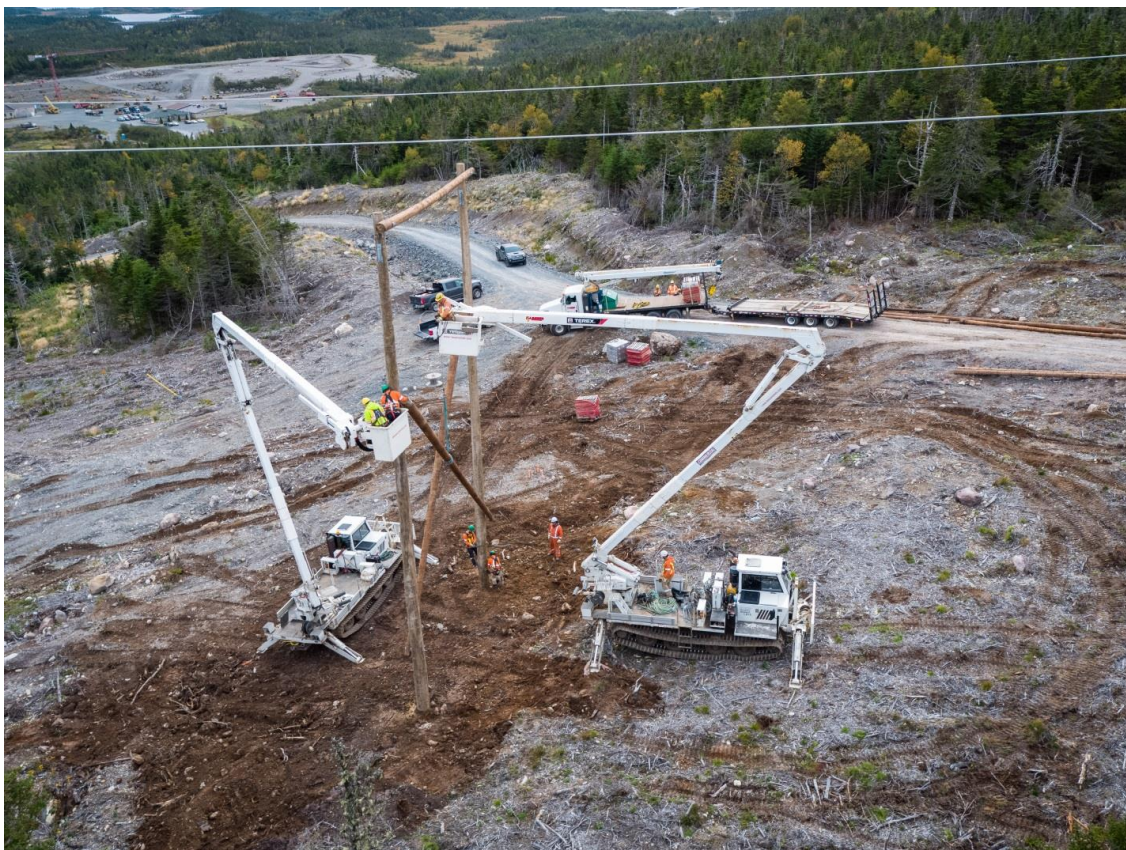
Figure 5 - Construction of Tangent ERS.
