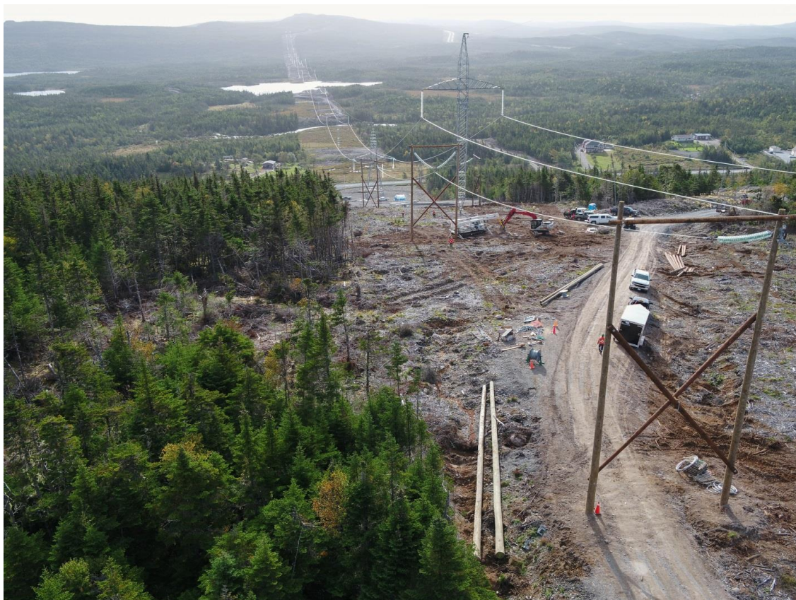
Figure 8 - Fully Strung and Completed Half Bypass.
