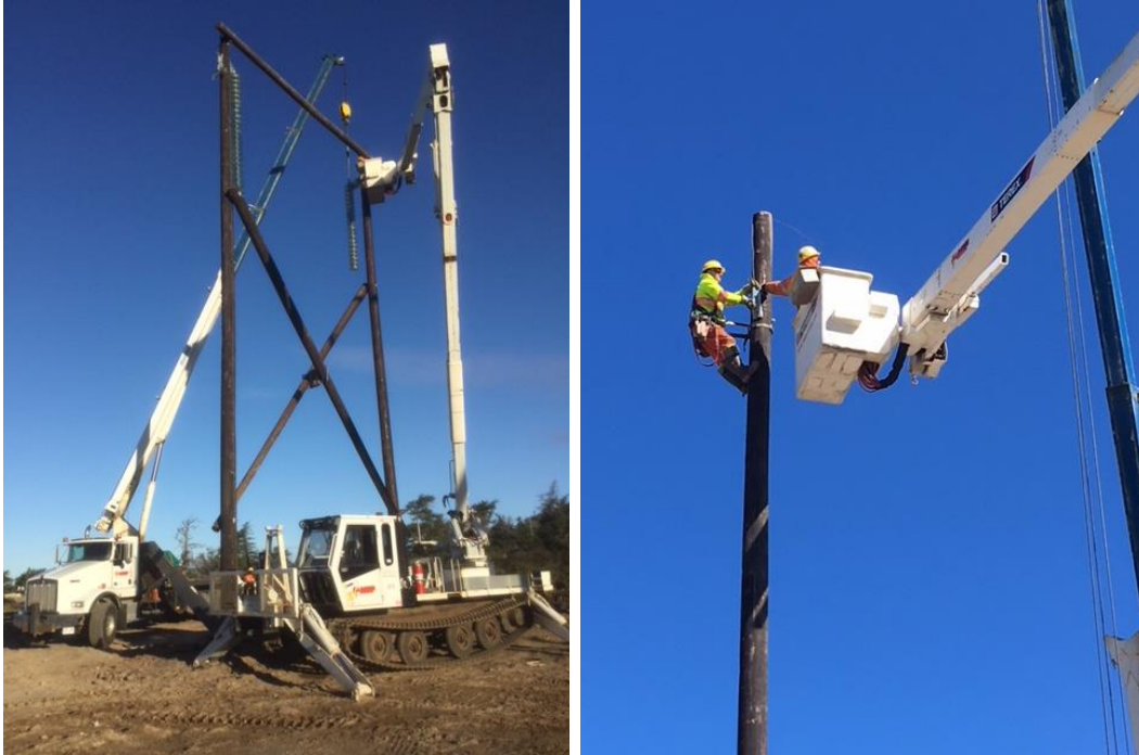
Figure 1- Wood Pole ERS Construction at SOP
